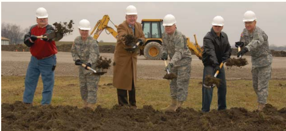
Participants in the Camp Perry Joint Use Training Facility ground breaking were (l. to r.) LTC Ralph Green, ARNG (Ret.), Deputy Post Commander; LTC Barbara Harrington-Clemmons, Installation Commander; Gary Anderson, Director of Civilian Marksmanship, CMP; BG Jack Lee, Deputy Commander, Joint Force Headquarters (Ohio), OH ARNG; Ken Clemmons, Camp Perry Base Engineer and COL Jim Chisman, Fort Ohio Installations Commander.
