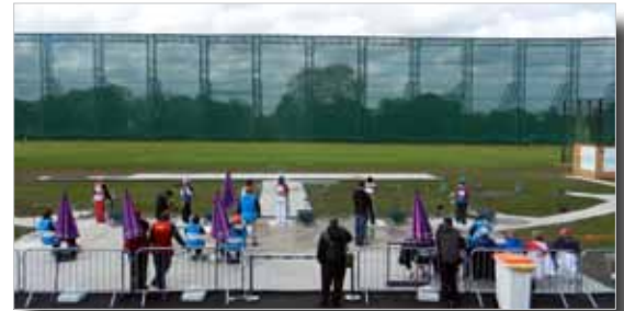
Skeet and Trap Ranges. The five shotgun events on the Olympic program will be contested on three combined skeet and trap ranges. The Shotgun Finals Range also has seating for 2,000 spectators. The shotgun ranges are enclosed on the front by an 89 foot high net to capture the fired lead shot.
