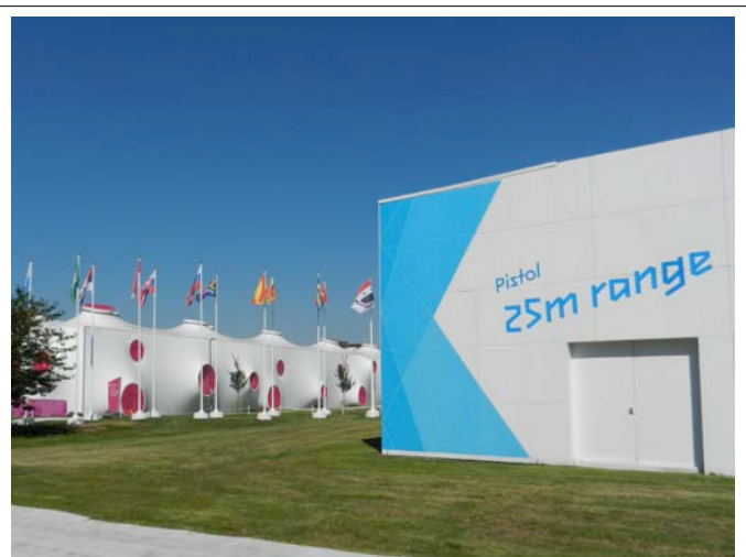
The exterior “Look” that was used for London 2012 venues produced what many regarded as the most attractive venue Olympic Shooting ever had.
